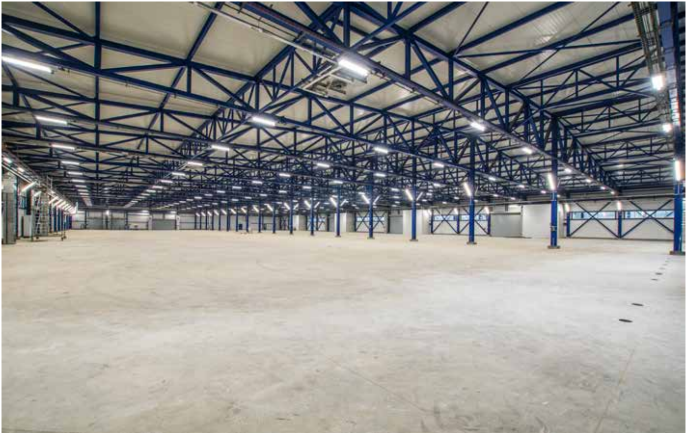
Nitrogen Plant. Puławy, Poland
